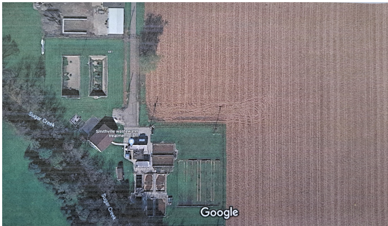
Figure 1. Study Site: Smithville Water Treatment Plant
