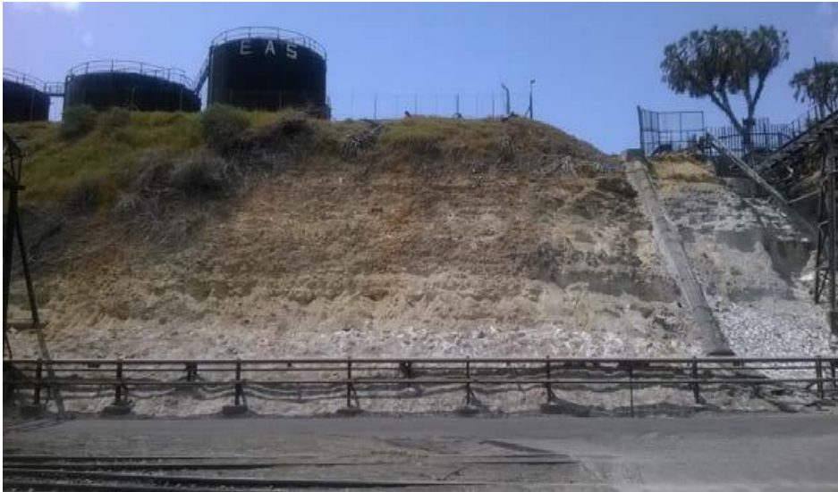
Figure 6: Showing evidence of discoloured vegetation around industries
