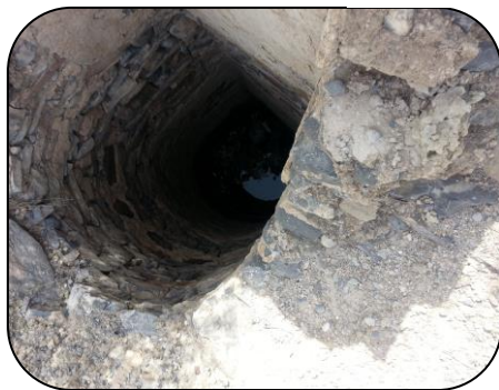
Falaj cleaning Channel
