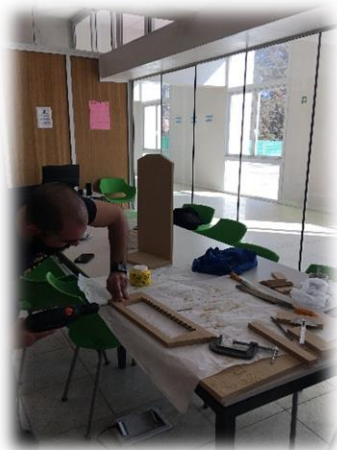
Image 13: Teacher Marianetti working on the construction of the shed.
