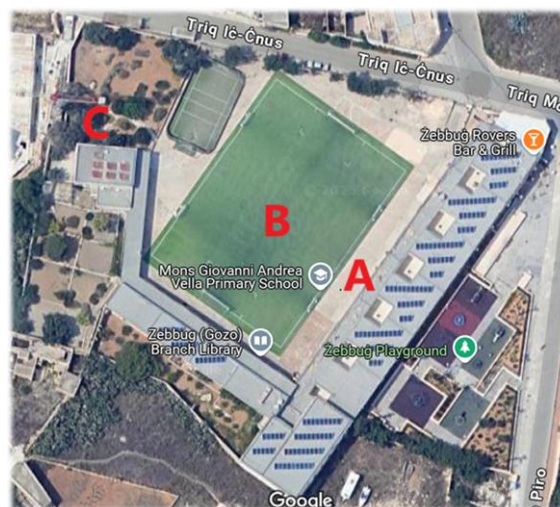
Figure 1 Study sites on an aerial view of the school
