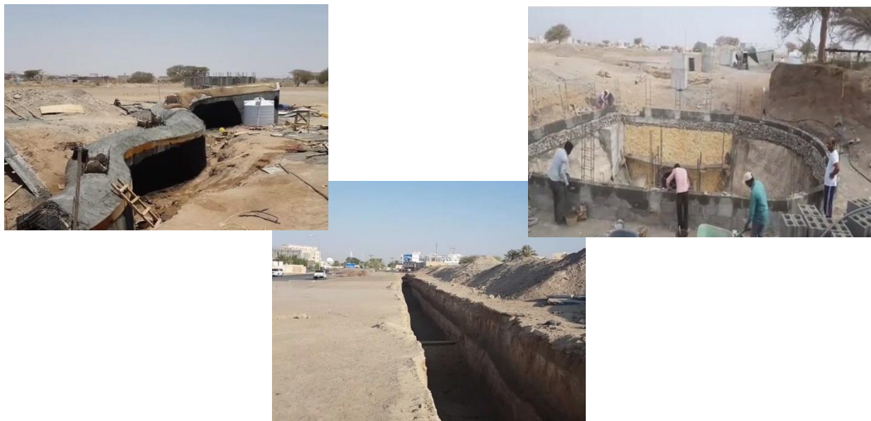
Maintenance works for the falaj
