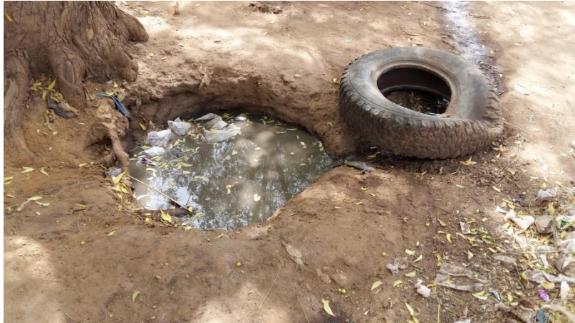
Figure 5: unprotected sump
