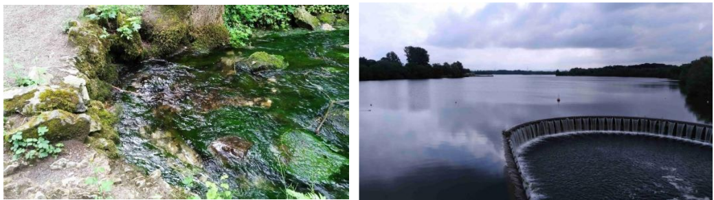
The rewilding and the ring around the Lippe river and the new way of the "Lippe" outside the lake in June 2024
